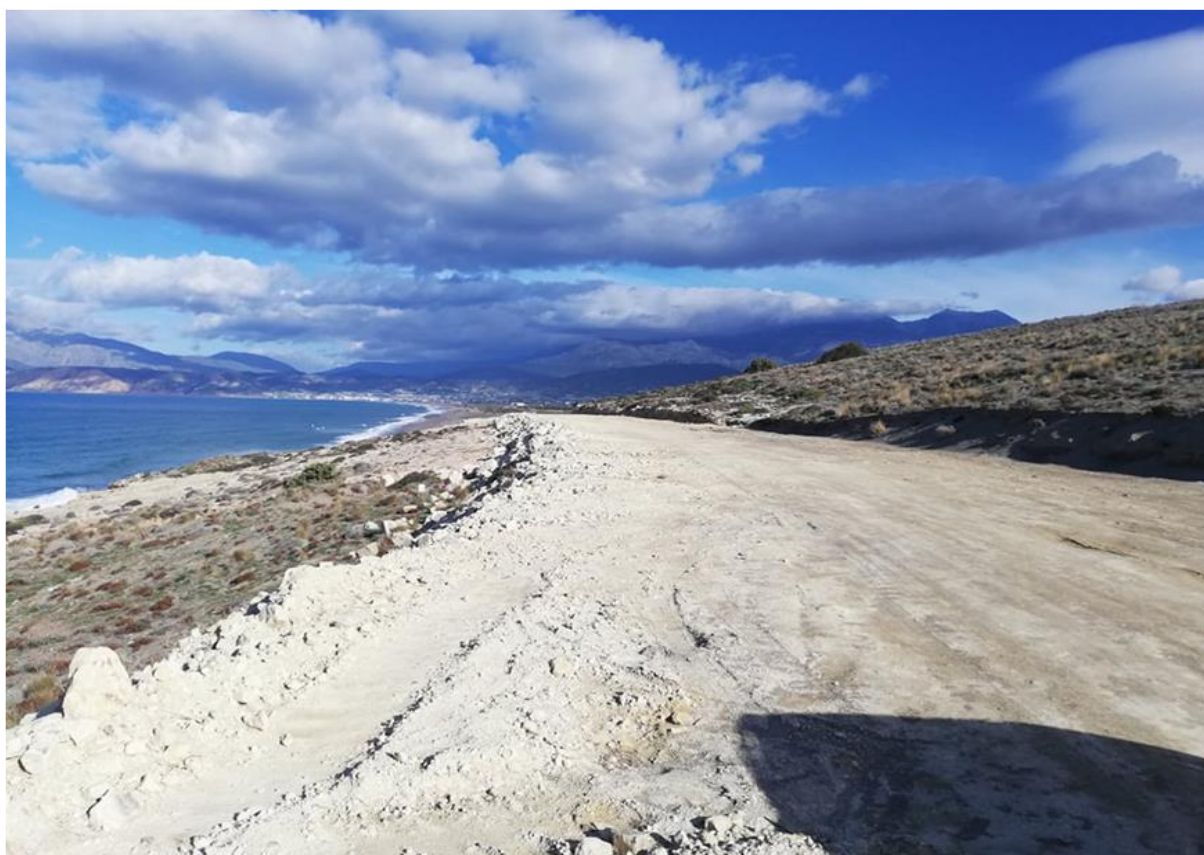
Picture of the road opened in Natura 2000 site (see case box that follows)
